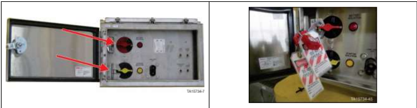
Battery isolation switch in OFF position with locks in place
