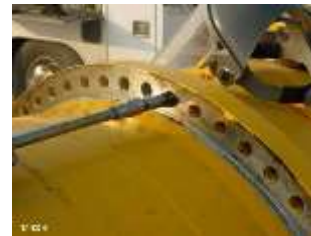
Cleaning paint and rust prior to torquing
